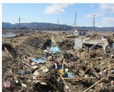
(c) 排水路の損壊
